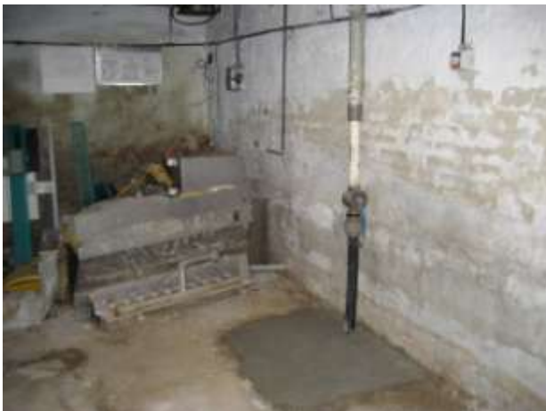
Heating system flood damage
