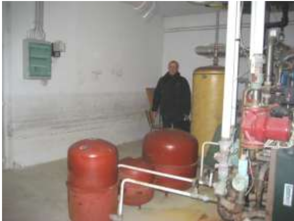
Picture of damage to equipment
